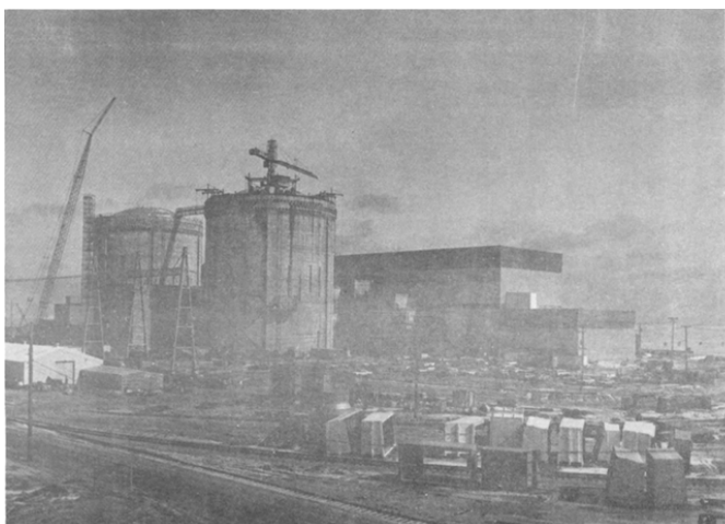
"Photo of Zion Construction Site Looking Northeast," AEC (January 1972) [3]
