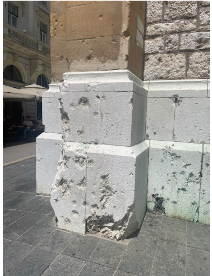
Figure 2: The Sacred Heart Cathedral in Sarajevo’s city center. While much of the building’s war damage has been repaired, bullet holes still chip away the cornerstone. Photograph taken by Evan Daneker.
